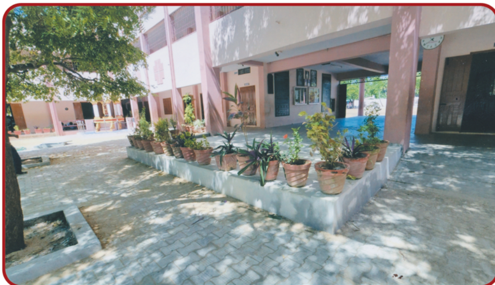
Laying Paver Blocks to Little Flower Higher Secondary School, Kumbakonam, under CSR Initiative
